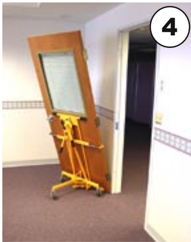
Align bottom corner of door with bottom corner of door jamb.
