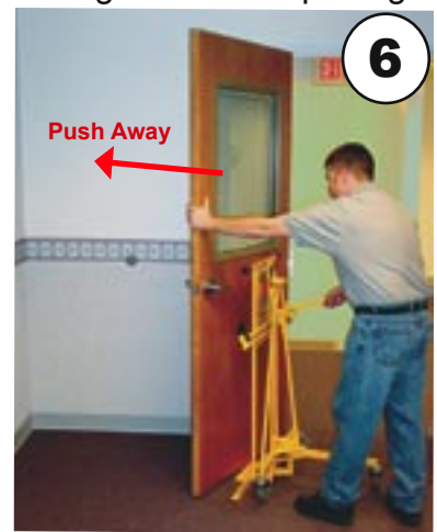
Fasten hinges to jamb or Door. After hinges are secured push door away from Doorminator™
